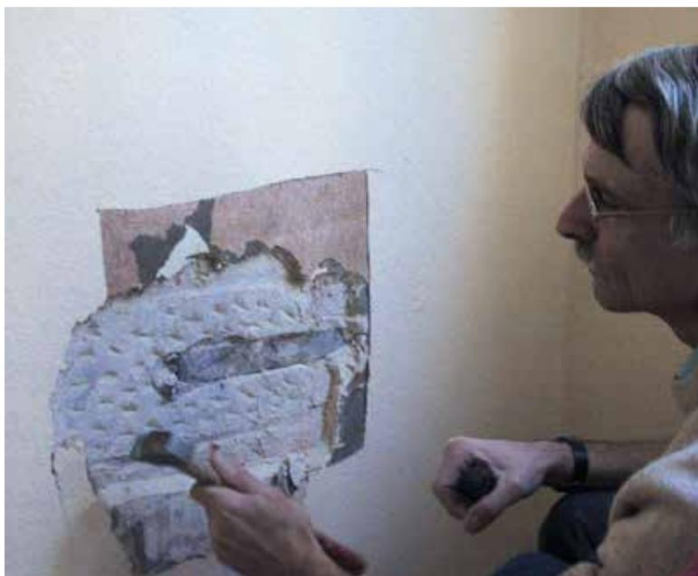
*L'Âne/Den Ezel*. A. Pien removing the render from a party wall to determine the shape of an anchor (© CHE, 2001).
