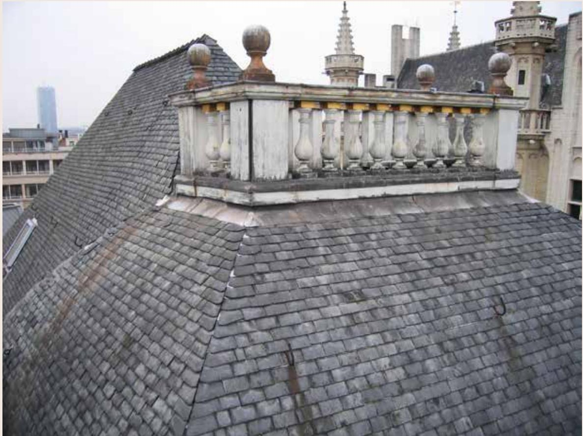
*Le Cygne/De Swane.* Wooden terrace on belvedere. Dislocated elements. Lower sections damaged. Widespread lack of maintenance (© HHU, 2008).
