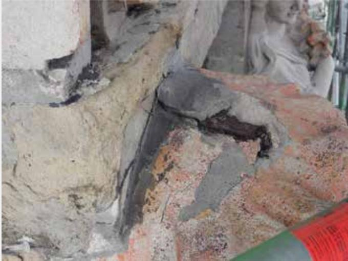
*Le Renard/De Vos.* Corrosion of a metal fixing pin at the top of a statue, causing it to fracture (© HHU, 2014).
