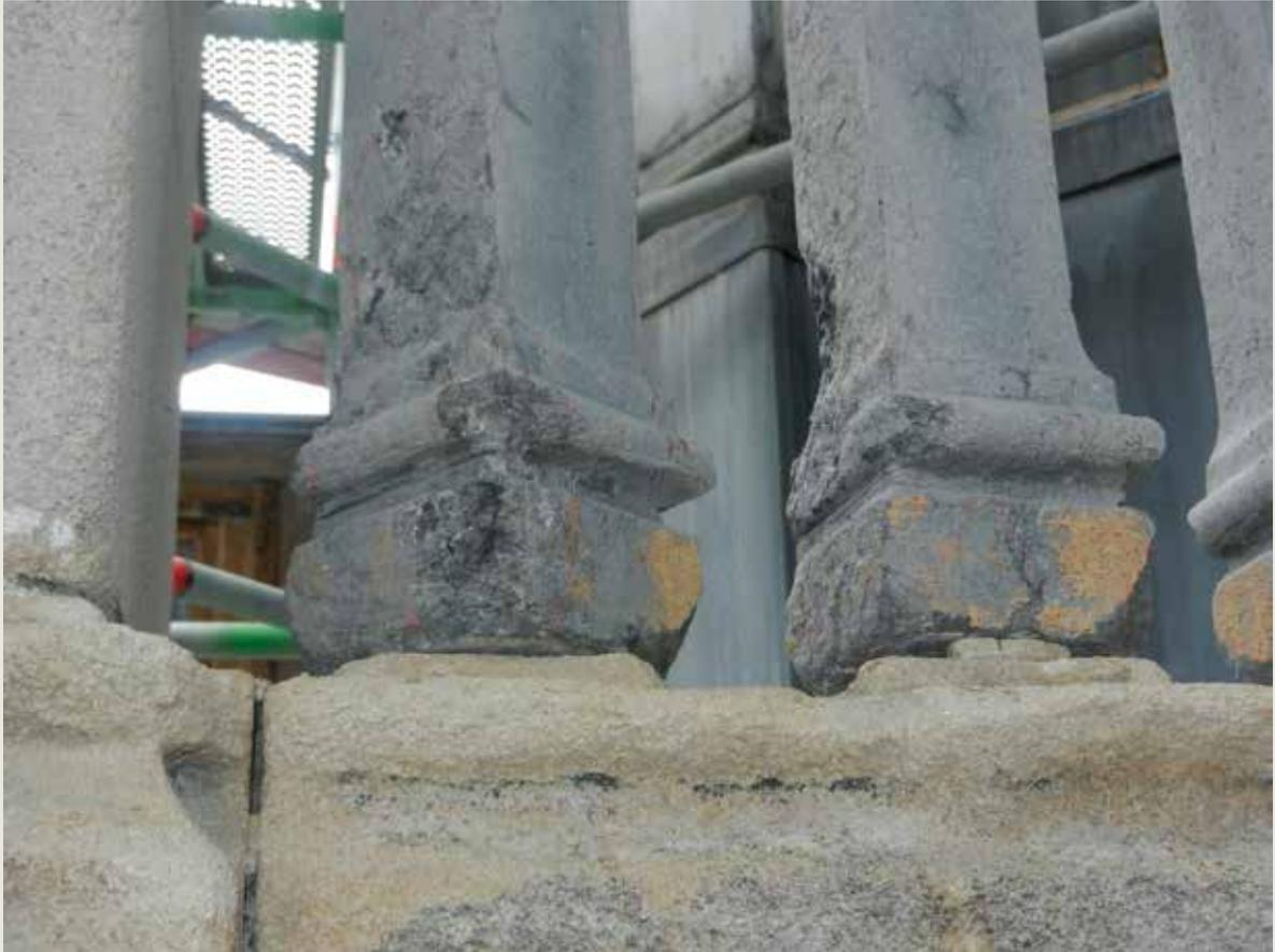
*Le Roi d'Espagne/Den Coninck van Spaignien. Pitting of the stone due to the presence of stylolites and the face-bedding of the stone in the balusters. Blue stone (© HHU, 2014).*
