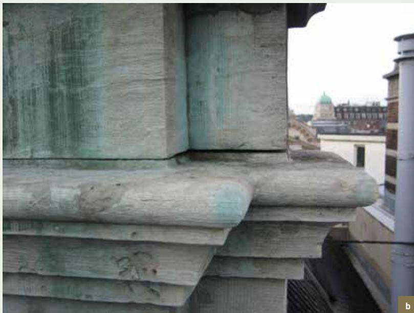
*La Brouette/Den Cruywagen*. Upper section of the façade. Green staining due to the oxidation of copper decorative elements. a) Overview; b) Detail of staining on the Gobertange stone (© HHU, 2014).
