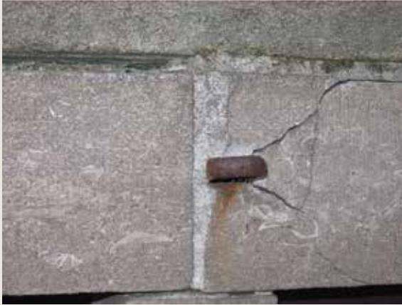
*Le Cerf/De Heert.* Cracks in a blue stone due to the rusting of the metal ring (© HHU, 2000).
