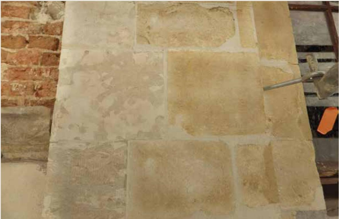
*Le Heaume/Den Helm* and *Le Paon/Den Pauw.* Detail of facing after cleaning showing the Gobertange stone facing (on the left) and the Balegem stone facing (on the right) on the façade of *Le Heaume/Den Helm*. The brick masonry on the façade of *Le Paon/Den Pauw* can be seen on the far left of the photo. This was revealed after the removal of loose render (© HHU, 2015).
