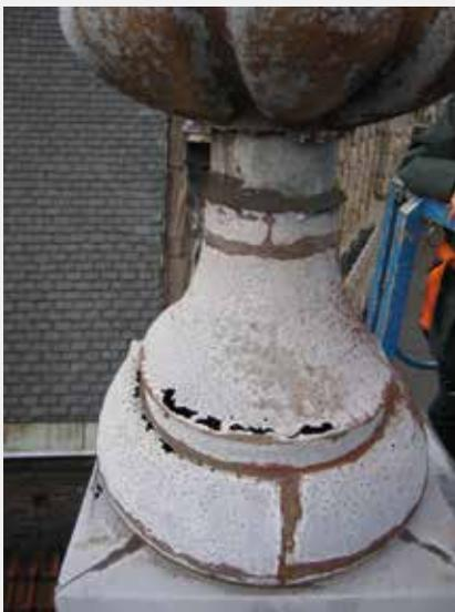
*La Rose/De Roose.* Detail of a corroded and pockmarked zinc vase (© HHU, 2000).
