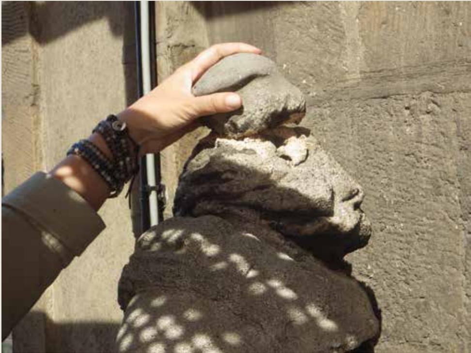
*Le Renard/De Vos.* Powdering of an Euville stone sculpted feature, causing the rupture of an element (© HHU, 2014).
