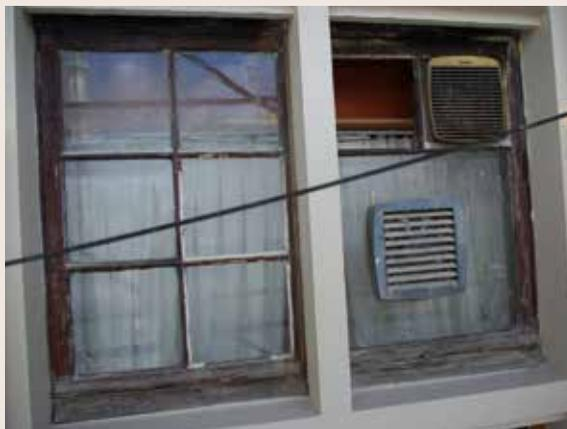
*La Chaloupe d'Or/De Gulden Boot.* Two window frames with damaged weatherboards and window sills. The frames were modified over time to incorporate ventilation outlets in a random fashion (© HHU, 2014).
