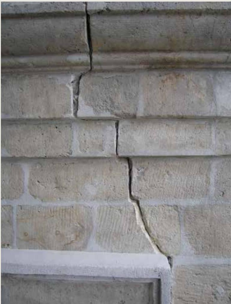
*Le Cygne/De Swane.* Crack in the original Balegem stone facing (© HHU, 2008).
