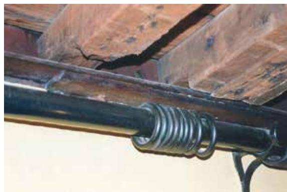
L'Ange/Den Engel - mezzanine, steel corner pieces bearing the old floor supporting structure (© HHU, 1999).
