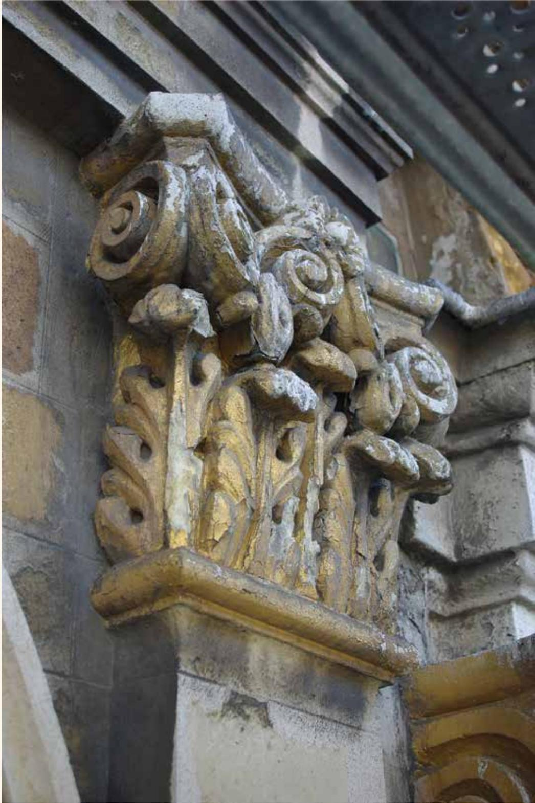
*Le Pigeon/De Duive*. Detail of a composite capital. Chipping of stone leading to damage to the gilding. General wear and tear of the gilding, build up of dirt (© HHU, 2012).
