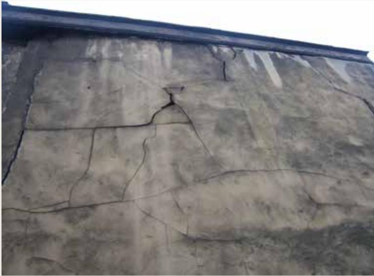
*Le Cygne/De Swane.* Delamination of the coating of the party wall, on the right (© HHU, 2008).
