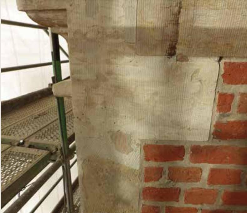
Side façade of the *Le Heaume/Den Helm* house. Detail of corner facing with Gobertange stone at the top and Balegem stone at the bottom and, on the right, brick masonry. Note the orange hue of the top stone due to the presence of iron in the glauconite contained in the stone (© HHU, 2014).
