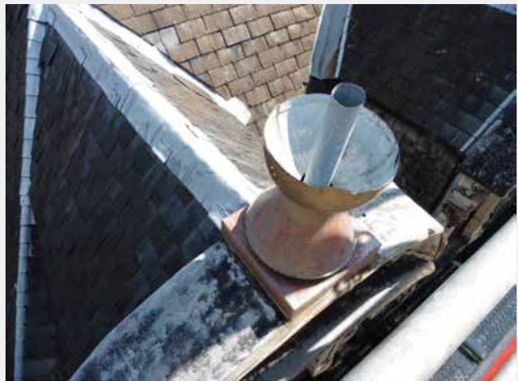
*Le Petit Renard et Le Chêne/Het Vosken en Den Eycke.* A vase split in two as a result of the corrosion of the zinc (© HHU, 2015).
