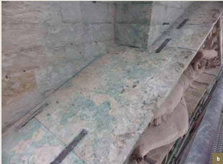
*La Louve/De Wolvin*. Detail of elements on the Gobertange stone pediment. Flaking. a) Front view with appearance of bioturbation on the stone; b) Top view of the pediment with flaking stone visible following the removal of the lead flashing (© HHU, 2014).
