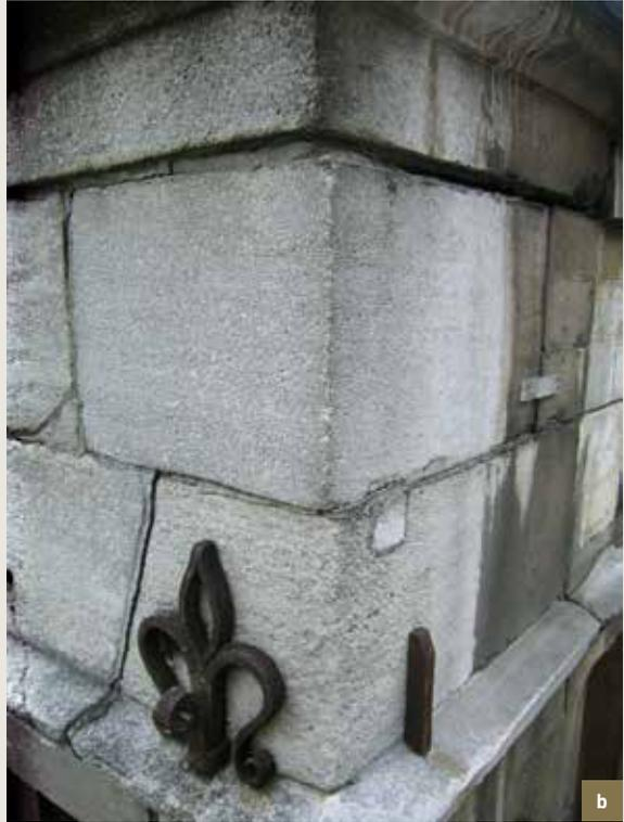
*L'Étoile/De Sterre.* a and b) Separation and open joints in the Euville stone as a result of structural problems (pressure from corroded metal elements in the floor) (© HHU, 2008).
