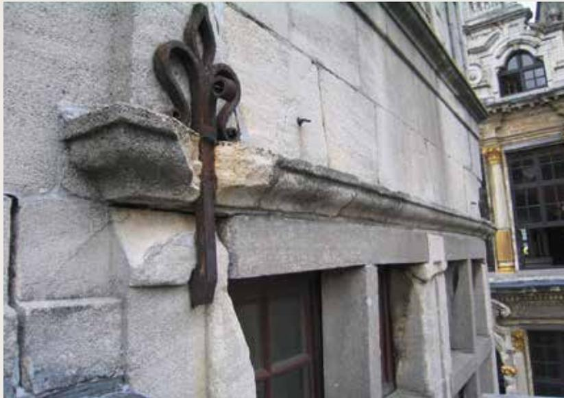
*Le Cerf/De Heert.* Euville stone exhibiting fracture caused by the corrosion of a metal anchor (© HHU, 2000).
