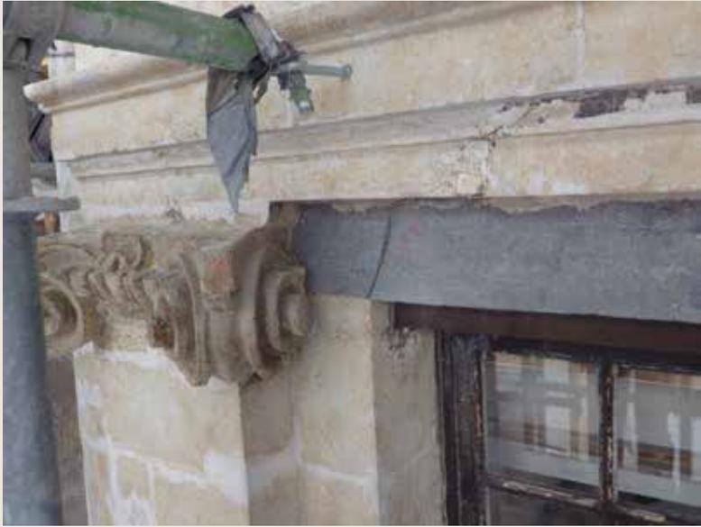
*Le Pigeon/De Duive*. Crack in the blue stone lintel caused by the development of rust on the metal lintel (© HHU, 2012).
