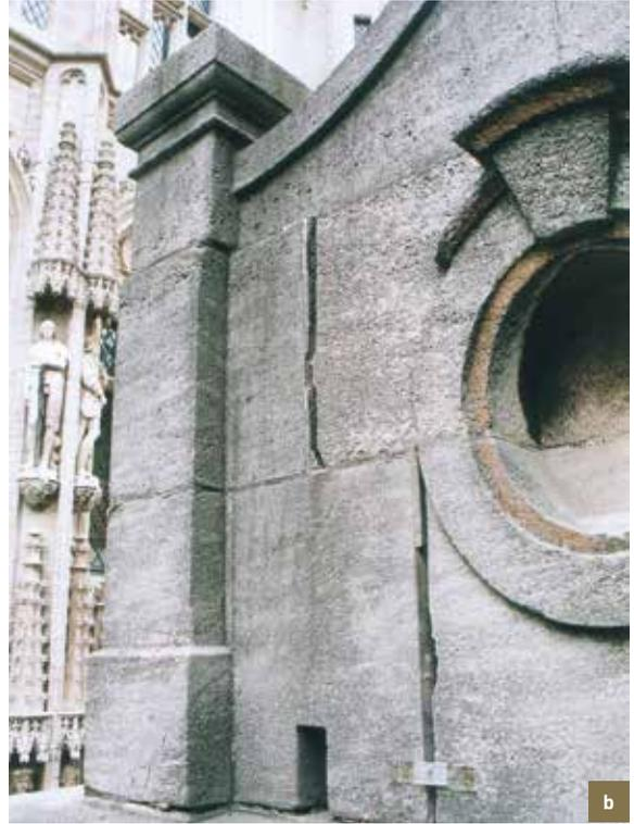
*L'Étoile/De Sterre*. Structural problems. a) Tilting of gable pediment on the façade facing the Grand Place. Euville stone; b) Separation of stones in the rear façade. Crack meter installed during the schedule of condition (© HHU, 2008).
