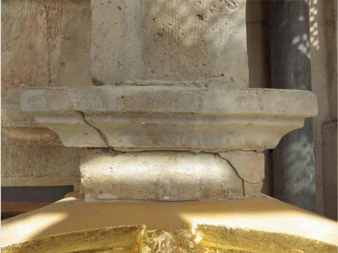
*La Brouette/Den Cruywagen*. Crack in the original Balegem stone facing (© HHU, 2014).
