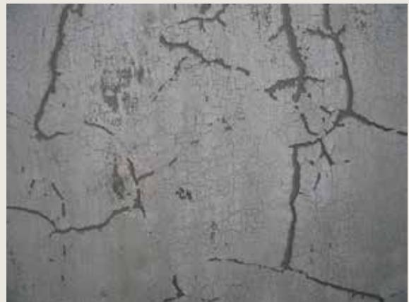
*Le Mont Thabor/Den Bergh Thabor.* Side façade. Cracking of the render and flaking of the paint (© HHU, 2014).
