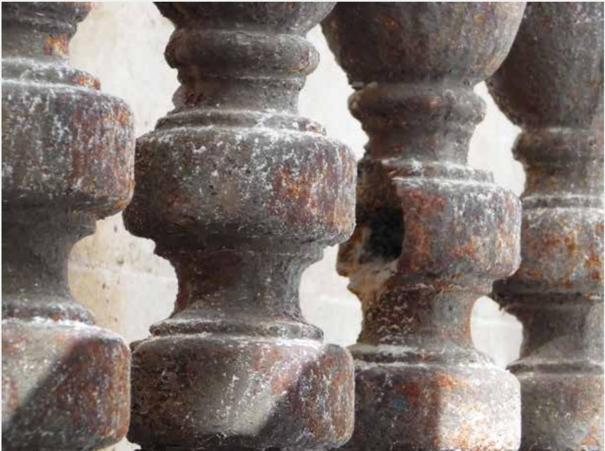
*Le Sac/Den Sack.* Corrosion of metal balusters, leading in some cases to the total degradation of material (© HHU, 2014).
