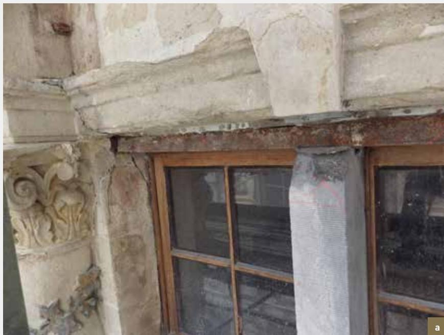
*La Brouette/Den Cruywagen.* Square metal bars dividing the lintels. The corrosion of the bars is causing the stone to fracture. a) Fracturing of elements made from blue stone and Balegem stone. Photographs taken during the restoration; b) Fracturing of an element made from Euville stone (© HHU, 2014).
