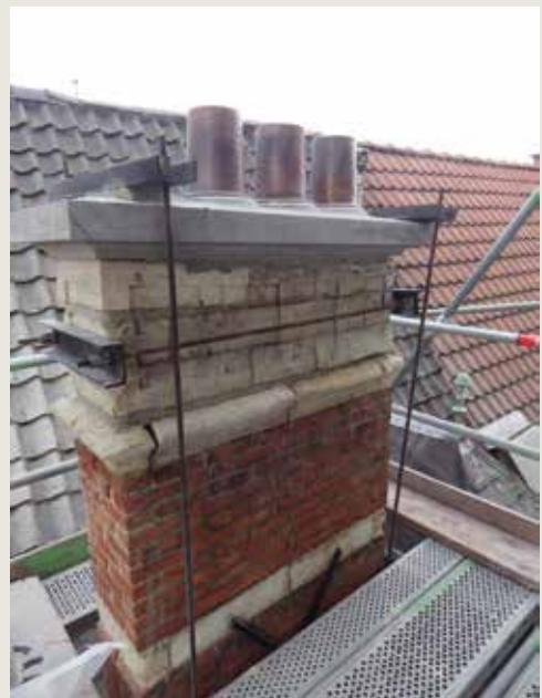
*Le Heaume/Den Helm.* Bracing of chimney after detection of instability (© HHU, 2000).
