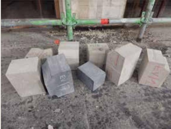
New stones delivered to the worksite to carry out the repairs required as a result of the chipping of stones due to corroding metal elements. Gobertange stone and blue stone (© HHU, 2015).
