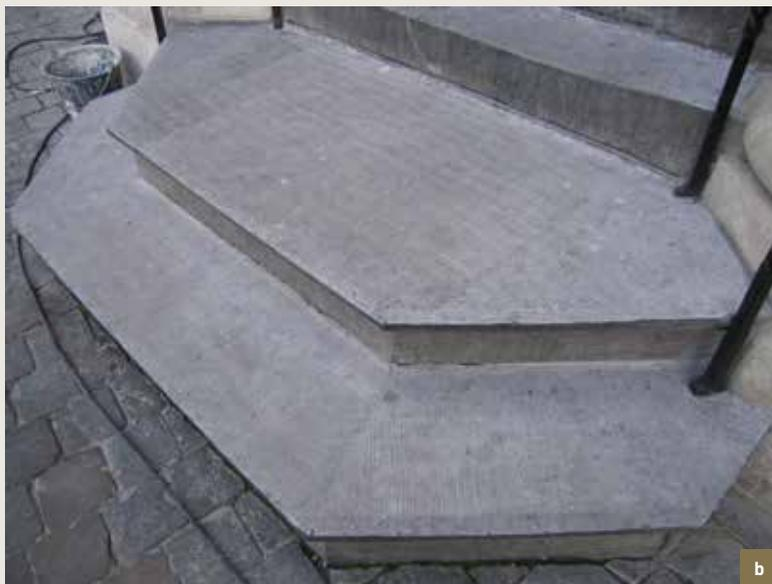
*Le Cygne/De Swane.* a) Chiselling of entrance steps in progress, based on the existing model. Blue stone; b) Finished job (© HHU, 2008).
