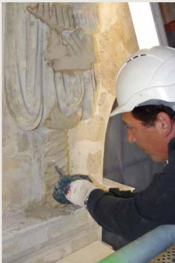
*Le Pigeon/De Duive*. Restoration in progress with smoothing mortar (twisted element of the mascarón). Unknown stone (© HHU, 2012).
