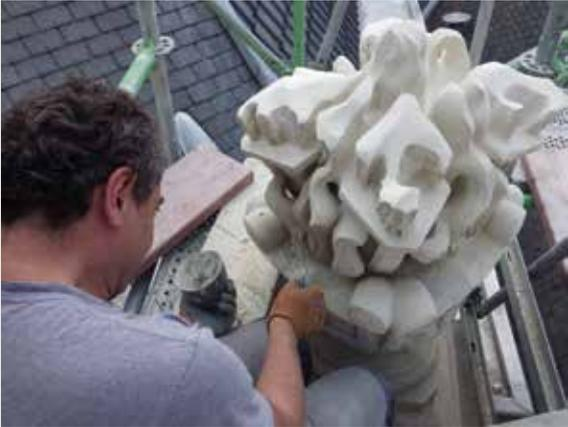
*La Louve/De Wolvin.* Flame finial on the pediment undergoing repair. French stone (© HHU, 2014).
