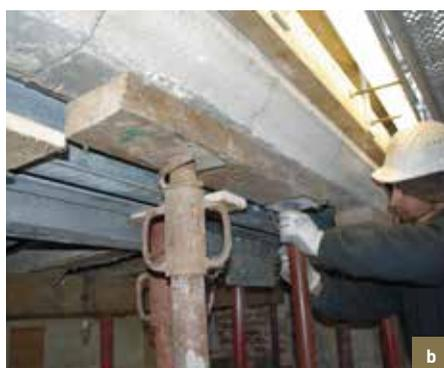
*Le Cerf/ De Heert.* a) Shoring of Euville masonry and fitting of metal clamp in order to remove the corroded metal beams; b) Installation of new galvanised steel beams (© HHU, 2008).
