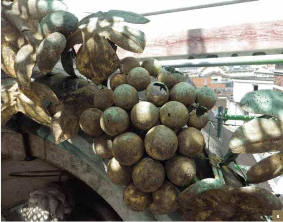
*La Brouette/Den Cruywagen.* Stages in the restoration of copper garlands. a) Condition before restoration (the bunches of grapes were badly corroded, some even having holes); b, c, d and e) Restoration in the workshop (with numbering), sanding with steel wool, cleaning with demineralised water and acetone, filling of holes (epoxy) and application of gilding (© HHU, 2014-2015).
