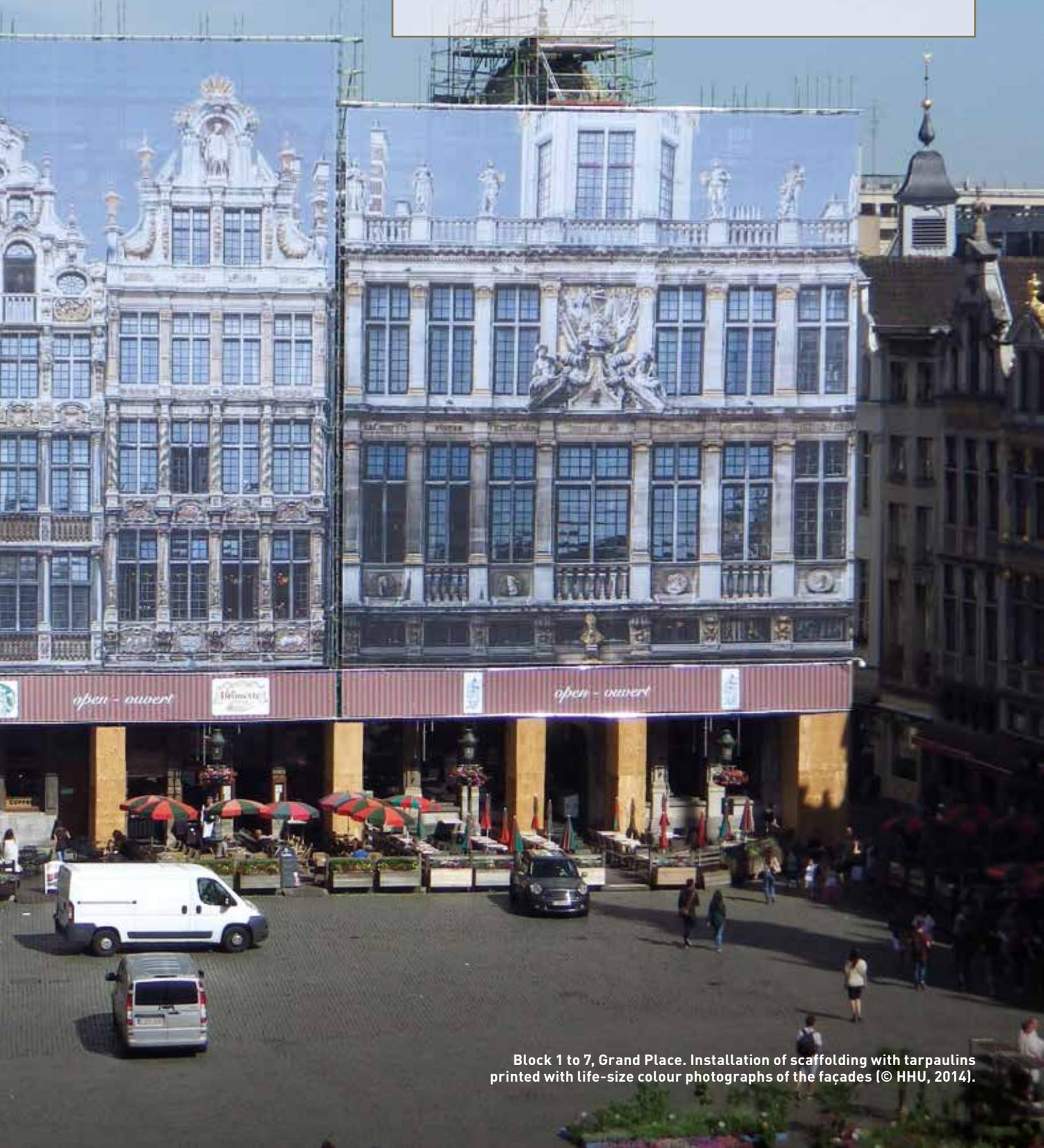
Block 1 to 7, Grand Place. Installation of scaffolding with tarpaulins printed with life-size colour photographs of the façades (© HHU, 2014).
