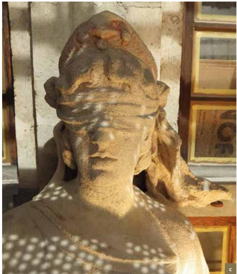
*Le Renard/De Vos*. Detail of the statue *La Justice/Justitia* (Pierre Comein, 1884). Euville stone. a) Before cleaning. Build up of dirt, peripheral crack on head; b) After cleaning; c) After the restoration of the stone (securing of the cracked head, patching with mortar using photographs of models) (© HHU, 2014-2015).
