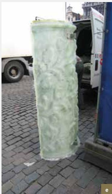
*La Maison des Brasseurs/Het Brouwerhuis. Column decorated with twisted foliage. a) The metal parts caused the element to crack or chip (cementing on original stone). Damaged state before casting and restoration; b) Core sampling of mortar; c) Moulding with silicone; d) Fibreglass-reinforced polyester resin shell; e) The cast is transported for possible reproduction; f) Finally, the elements were restored *in situ*, painted and gilded (© HHU, 2014-2015).*
