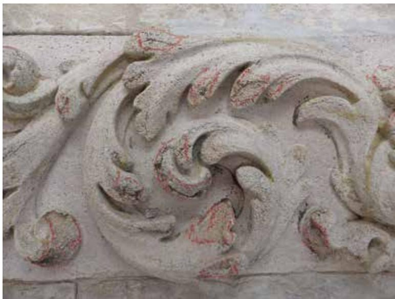
*La Brouette/Den Cruywagen. Detail of scrollwork with red chalk marking the parts to be repaired with smoothing mortar. Euville stone (© HHU, 2014).*
