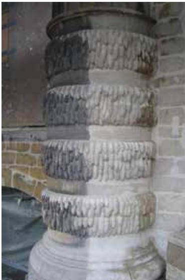
*La Maison des Brasseurs/Het Brouwerhuis*. Cleaning test. Detail of rustic bossages on columns. Balegem stone. Low pressure hydro-pneumatic swirling vortex technique (© HHU, 2004).
