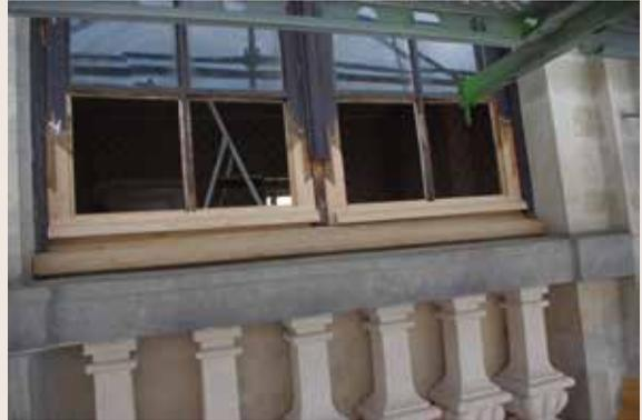
*Le Pigeon/De Duive*. Replacement of sill and weatherboard and fitting of grafts. Oak wood (© HHU, 2008).
