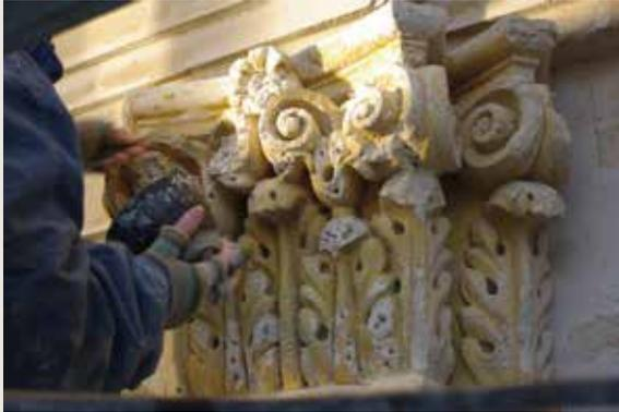
*Le Pigeon/De Duive.* Detail of two capitals undergoing repair. Unknown stone (© HHU, 2012).
