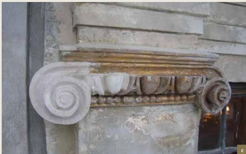
*La Rose/De Roose.* First floor, volute on a capital undergoing restoration: a) Integration of a Massangis stone graft; b) Sculpting in progress; c) Finished element (© HHU, 2008).
