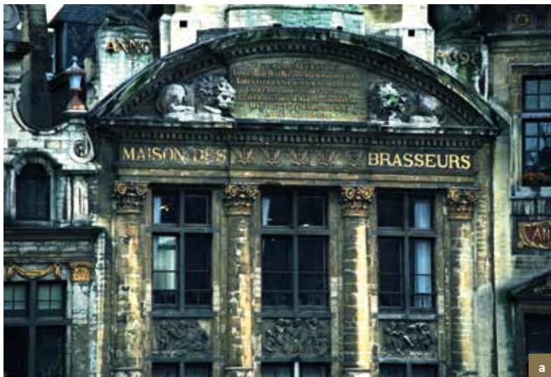
*La Maison des Brasseurs/Het Brouwerhuis*. a) Condition before restoration: biological growth (moss), dirt and black crust (atmospheric pollution), metal oxide stains, etc. (© HHU, 2000); b) Condition after restoration (© Utopix, M. Ploton, 2018).
