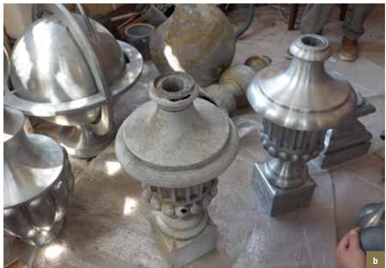
*Le Sac/Den Sack. Zinc vase.* a) Cracked and pockmarked original element; b) Old and new elements (© HHU, 2014-2015).
