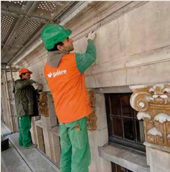
L'Étoile/De Sterre. Repointing with mortar (© Daylight, 2008).
