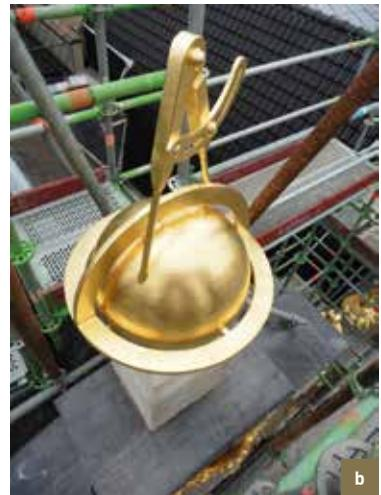
*Le Sac/Den Sack. Globe.* a) Archive drawing that was used for the creation of the new zinc globe, due to the existing globe being too badly damaged (© AVB); b) New gilded globe on the apex of the gable (© HHU, 2014-2015).
