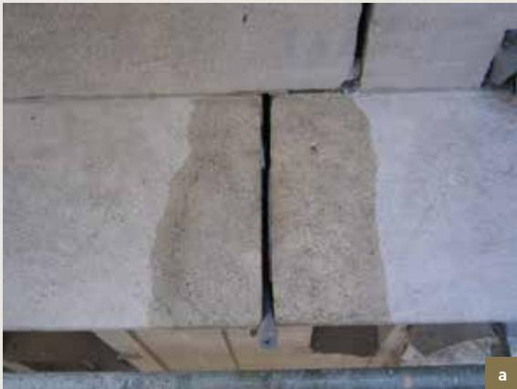
L'Étoile/De Sterre. a and b) Injection of grout (© HHU, 2008).
