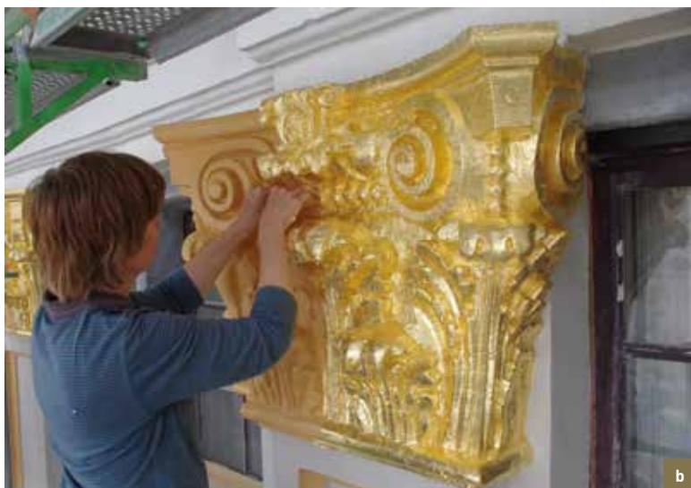
*La Chaloupe d'Or/De Gulden Boot.* Detail of a capital. a) Checking the gilding chosen; b) On the left: orange-yellow preparatory base layer. On the right: application of gold leaf on mixtion (© HHU, 2012).
