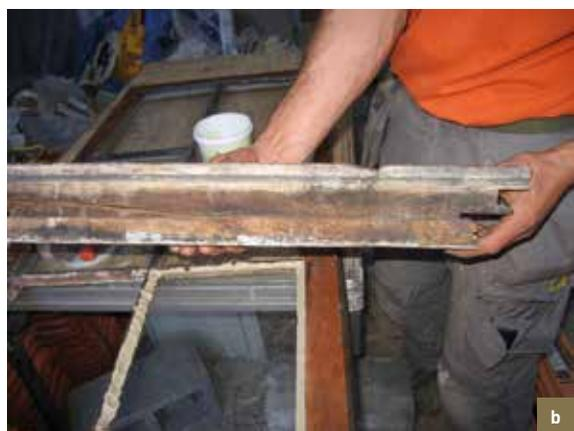
*La Rose/De Roose. Damaged oak wood pieces. a) A weatherboard (lower part of window frame) requiring replacement; b) A window sill requiring replacement (© HHU, 2014).*
