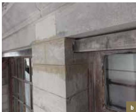
*Sainte-Barbe/Sint Barbara.* a) Detail of the stone to be replaced, marked with a cross using red chalk; b) New Gobertange stone elements and stainless steel bars (© HHU, 2015).
