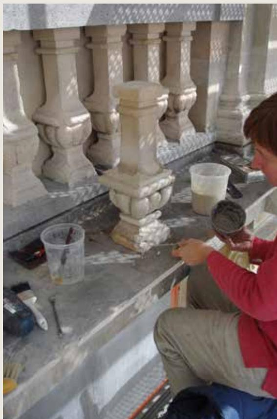
*Le Pigeon/De Duive*. Detail of a baluster undergoing restoration and repair with smoothing mortar. Marble type Euville stone (© HHU, 2012).
