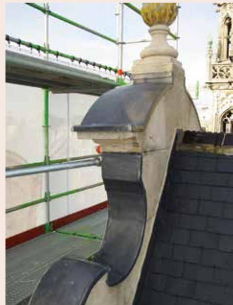
*Aux Armes de Brabant/De Wapens van Brabant*. Restored lead on parts of gable exposed to rainwater runoff (© HHU, 2008).
