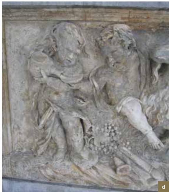
*La Maison des Brasseurs/Het Brouwerhuis*. Details of one of the apron panels on the 2<sup>nd</sup> floor depicting the harvest (Pierre Van Dievoet, 1698). Most likely Avesnes stone. a) Build-up of dirt on sculpted *putti* prior to restoration, with partial cleaning on the left; b) Application of compresses composed of an ammonia-based cellulose paste to soften the black crust; c) Finalising cleaning using a micro-sandblaster; d) Condition after cleaning (© HHU, 2004).
