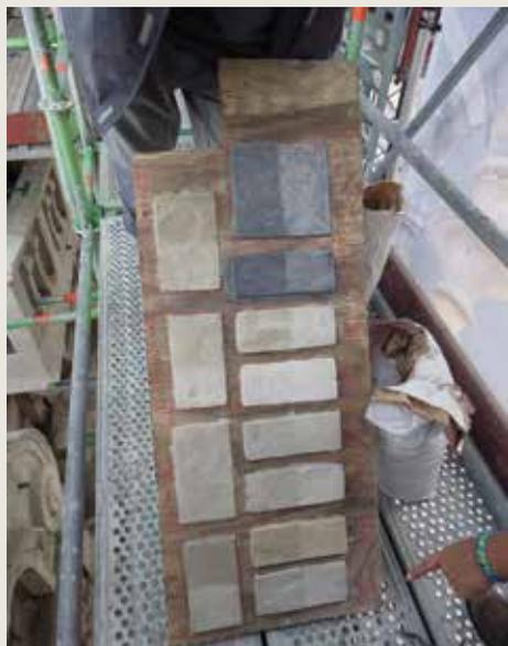
Samples of smoothing mortar created for comparison with the stones to be repaired and to choose the texture, grain size and colour. This palette of samples is kept on the site at all times (© HHU, 2014).
