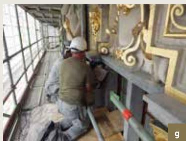
*Le Sac/Den Sack.* Stages in restoring a capital: a) Damaged condition; b) Removal of element; c) Moulding of a capital in good condition; d) Silicone mould with fibreglass-reinforced polyester shell; e) Plaster positive; f) New sculpture made from Savonnière stone; g) Integration of the stone element (© HHU, 2014-2015).
