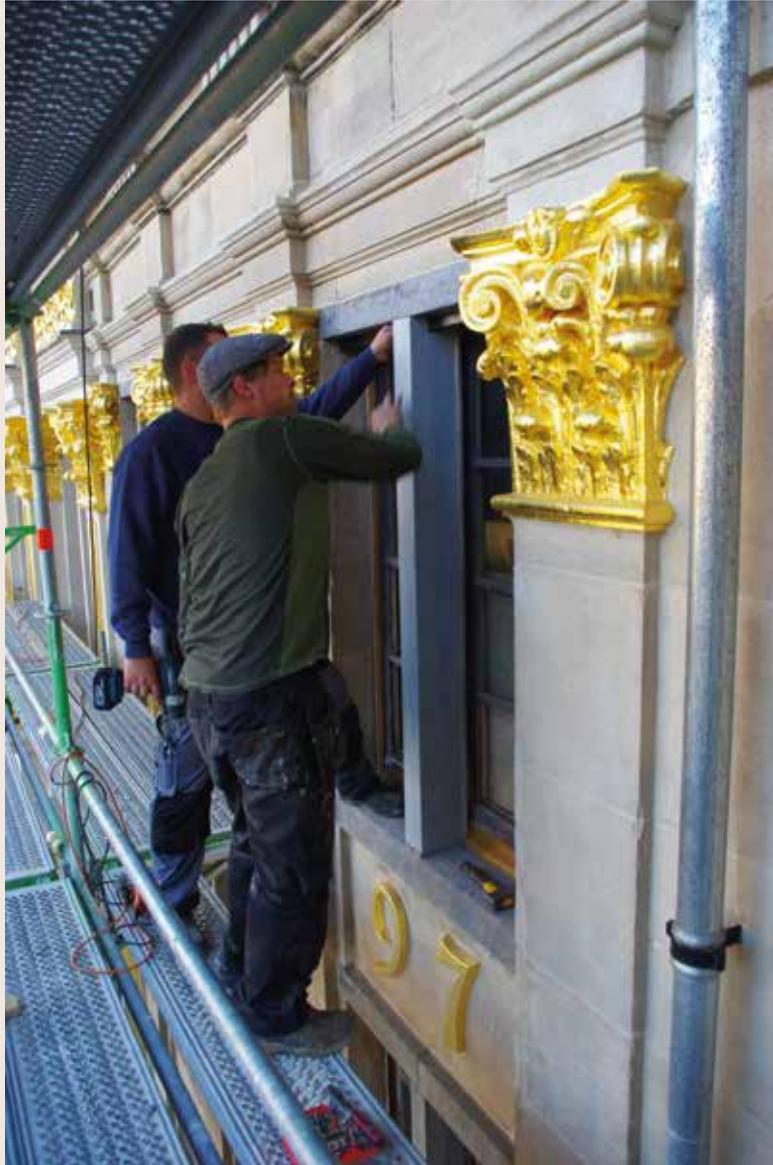
*L'Ange/Den Engel.* Installation of imitation blue stone mullions made of wood. They can be dismantled to facilitate removals (© HHU, 2008).
