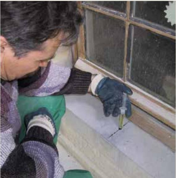
L'Âne/Den Ezel. Blue stone threshold. Injection of product (two-component epoxy) via small holes prepared for this purpose (© HHU, 2003-2004).
