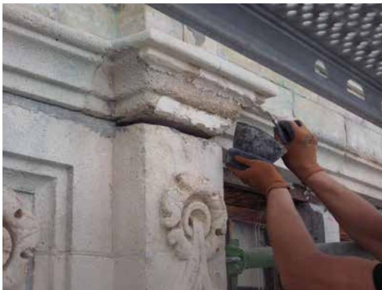
*La Brouette/Den Cruywagen. Mouldings undergoing restoration and repair with smoothing mortar. Euville stone (© HHU, 2014).*
