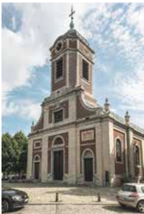
Sint-Pieterskerk in Ukkel, 1778-1782, arch. J.-F. Wincqz. (A. de Ville de Goyet © GOB)
